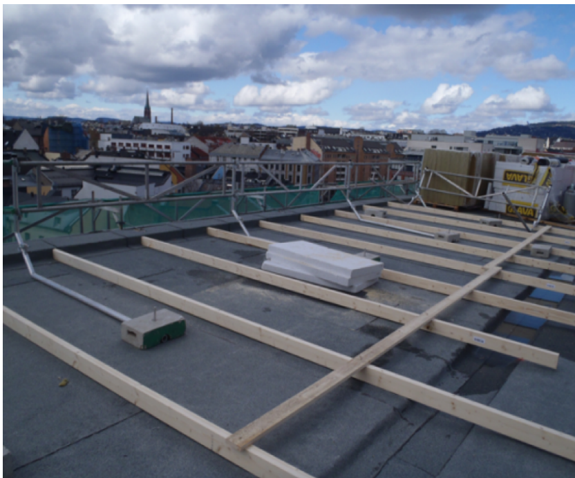
Picture 2 - secure of edges by removable railing
