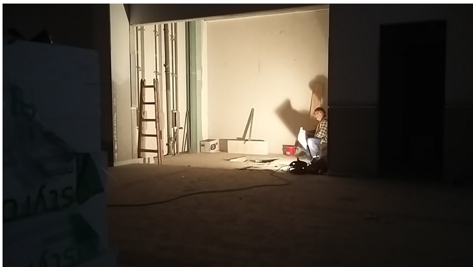
Picture 16 - part of safe work is rest
