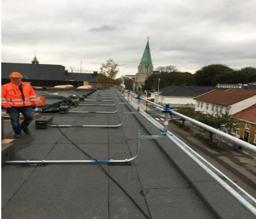
Picture 1 - secure of edges by removable railing
