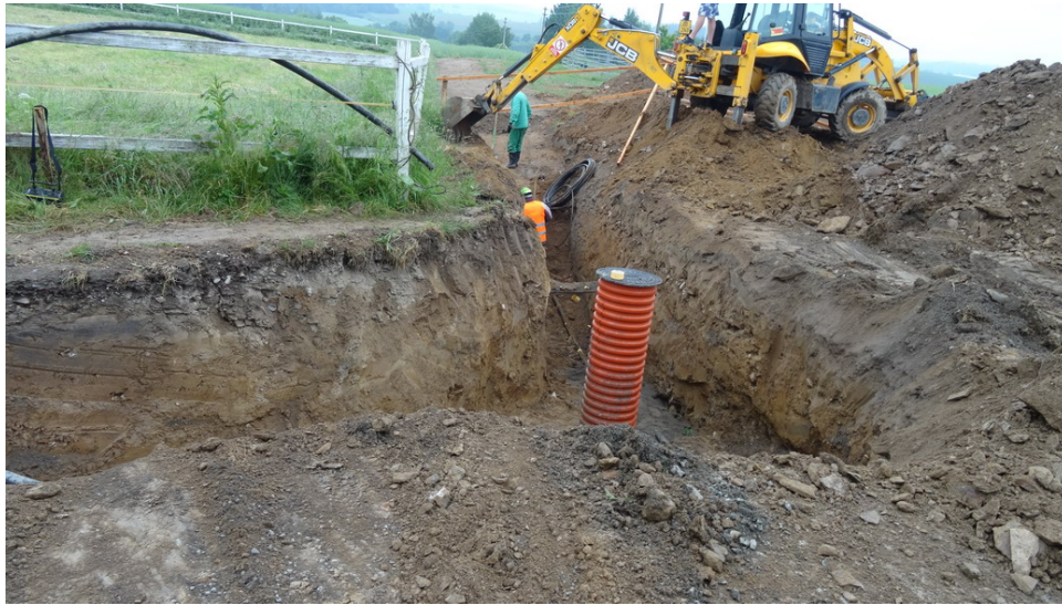
Picture 17 - working in excavation under the working machine
