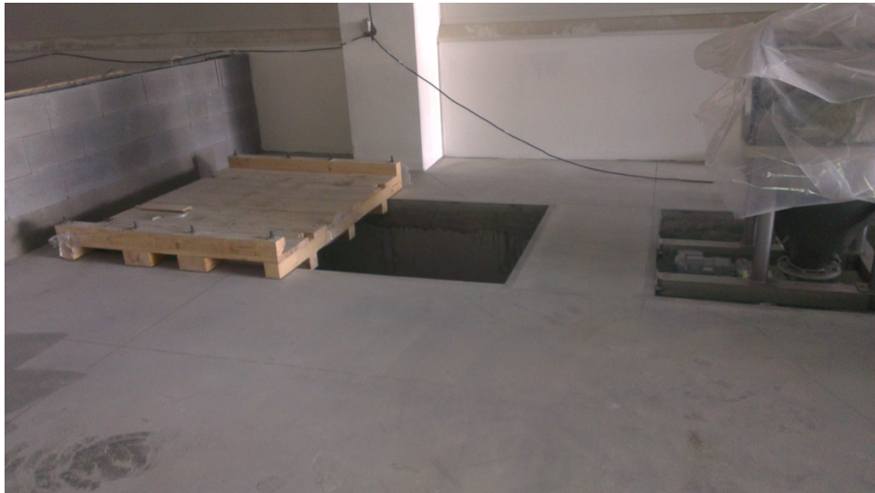
Picture 18 - uncovered hole
