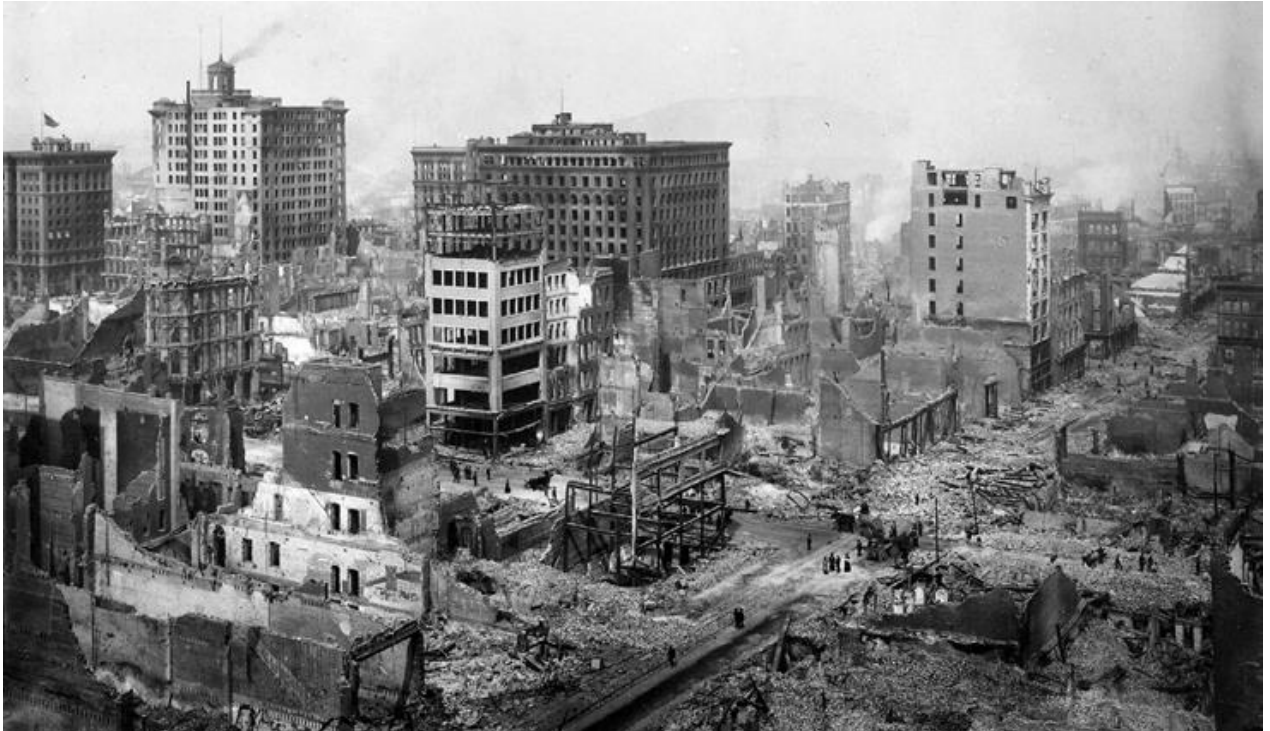
Figure 1 Steel frames performance in The 1906 San Francisco Earthquake (National Archives & Records Administration).
