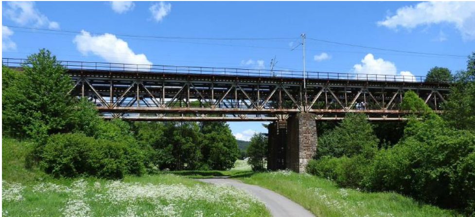
Figure 48. TU 2362 Bridge. Ref. [16]
