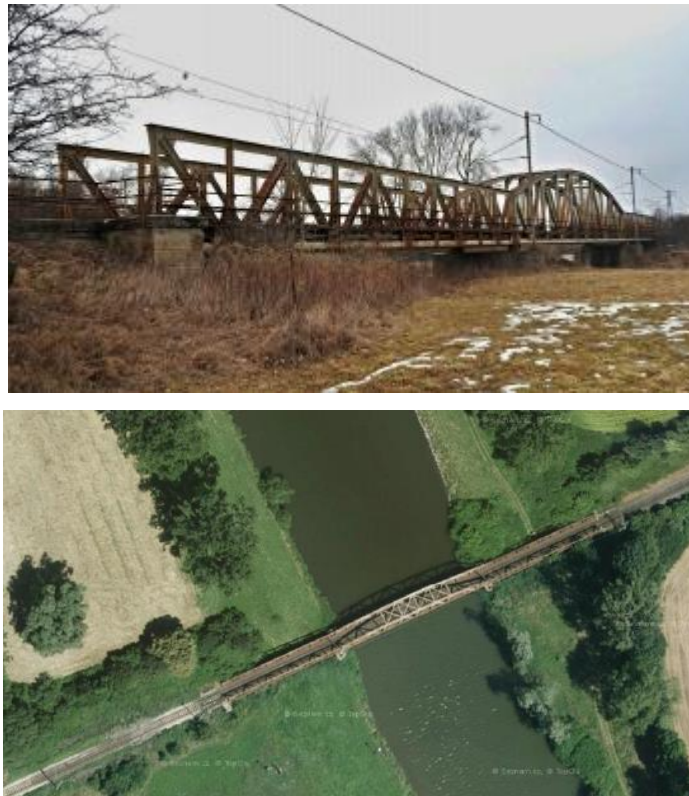
Figure 36. TU 2101 Bridge. Ref. [16]
