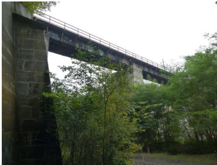
Figure 31. TU 581 bridge. Ref. [16]
