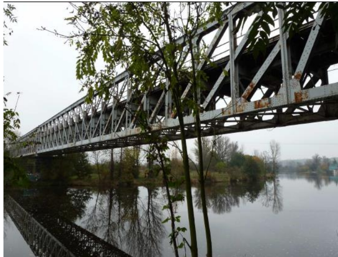
Figure 27. TU 502 bridge. Ref. [16]
