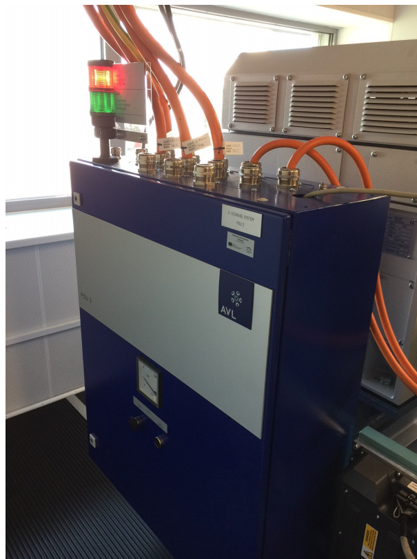
Figure 5.5. PDU unit of the battery simulator
