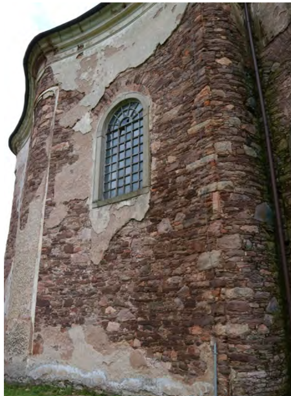
Figure 4.1. Enclosure wall masonry from the exterior shows non-uniform mixture of stones making up the outer leaf masonry layer
