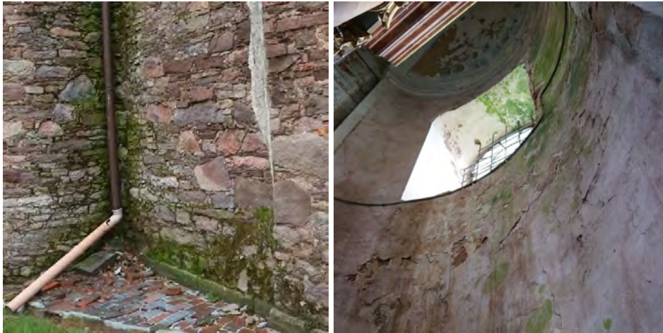
Figure 3.6. Biological growth at the kink at the lateral façade where a water downpipe is located from the exterior (left) and the interior (right)
