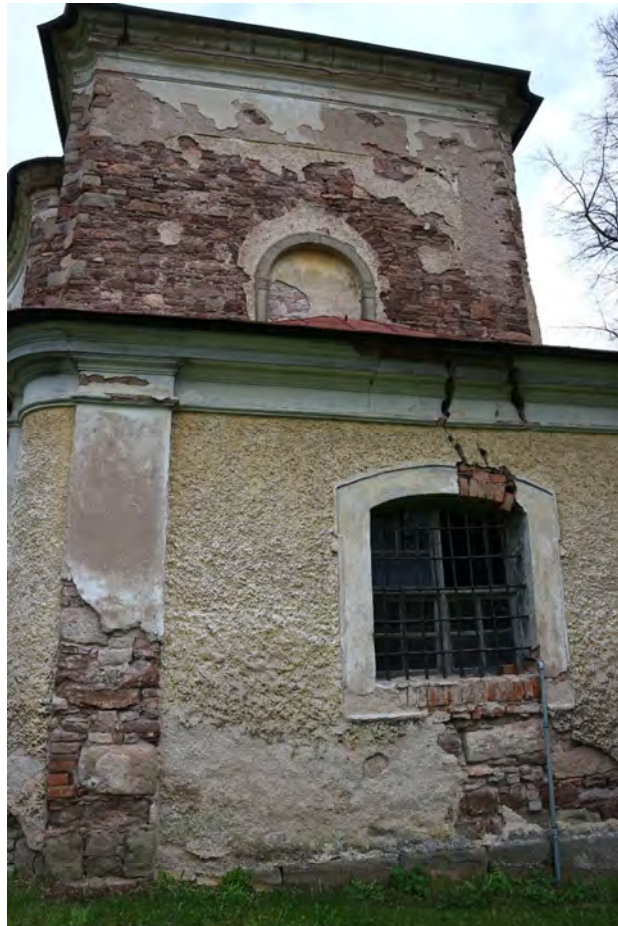
Figure 3.11. Large crack on the western facade behind the sacristy
