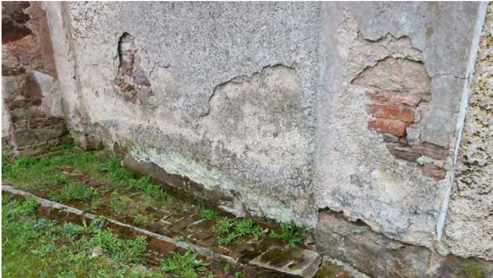
Figure 3.12. Ill-located brick blocks showing signs of reckless repair
