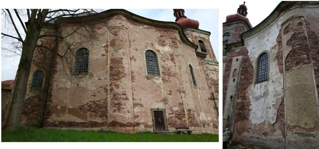
Figure 3.7. Render and plaster deterioration on the external southern wall (left) and northern wall (right)
