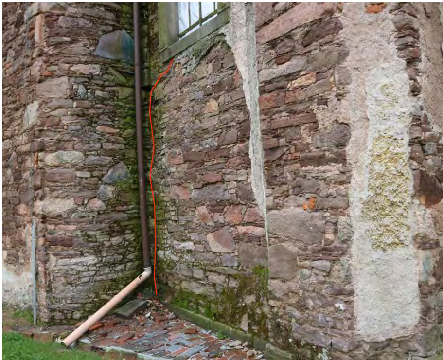
Figure 3.10. Crack on the longitudinal façade near the kink of the church
