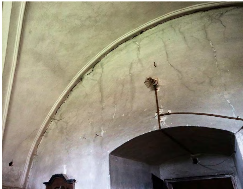
Figure 3.9. Continuous crack separating the sacristy vault to the main church wall
