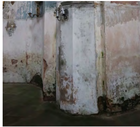
Figure 3.3. Moisture signs in church interior
