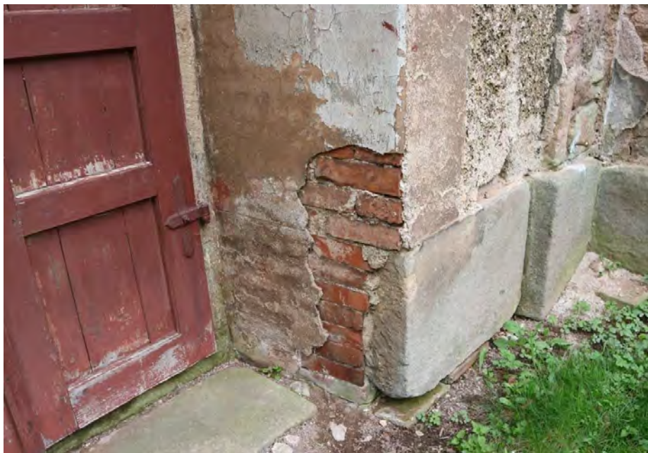
Figure 3.13. Frame around sacristy door
