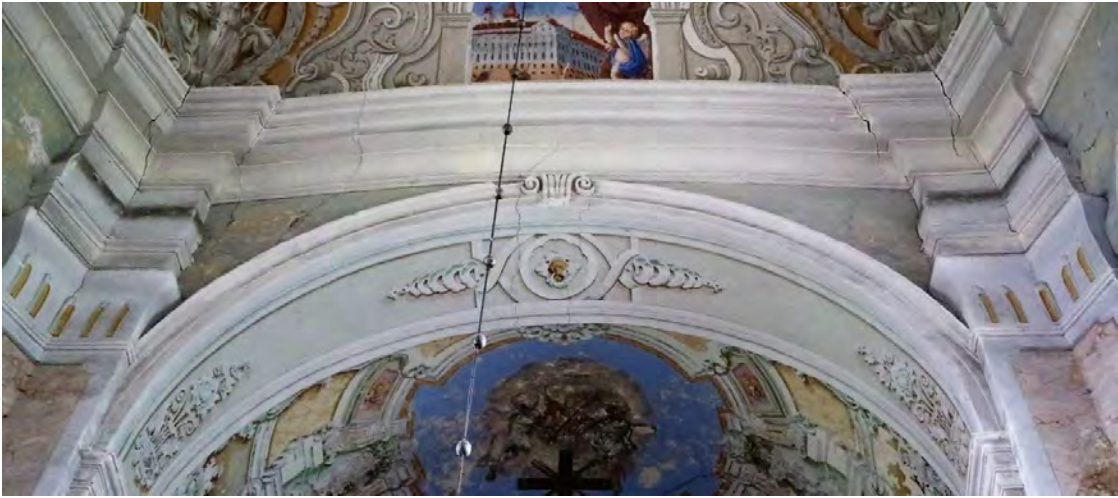
Figure 3.8. Cracks on transverse arches bridging the northern and southern facade
