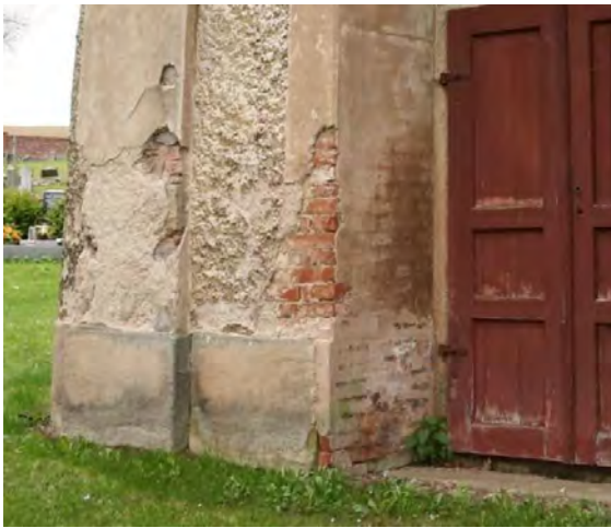
Figure 3.2. Moisture signs at the church exterior
