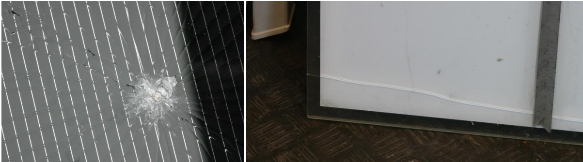
Fig. 19: Front glass damage caused by the stone and back glass damage caused by edge punch
