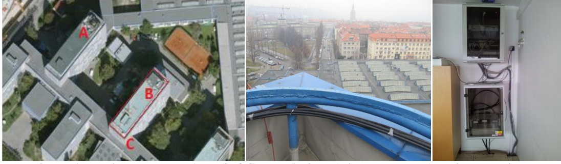
Figure 1. Testing polygon: a) roof of CTU building b) Alcatel cable c) optical terminal
