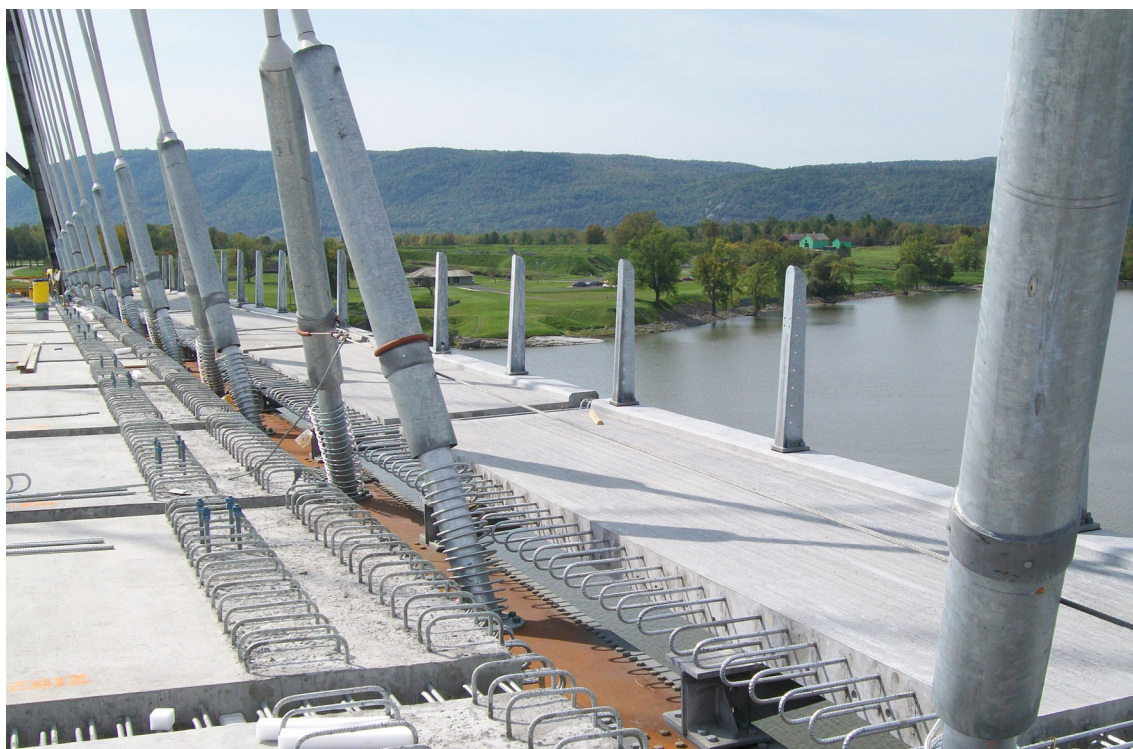
Obr. 6 Lake Champlain Bridge Project, New York (9)
