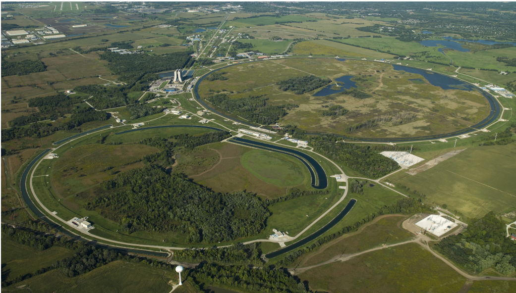
Figure 1.6: The Fermilab overview (Author: Fermilab)
