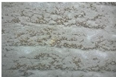
Obr. 76: Detail textury betonu [29]
