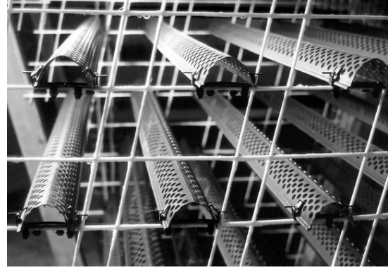
Figure 2.6 Splash fill V-bar [18]
