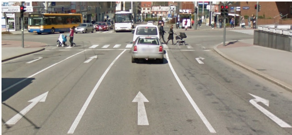
Figure 4.2: Horizontal Road Marking in Zlin, Czech Republic [52]
