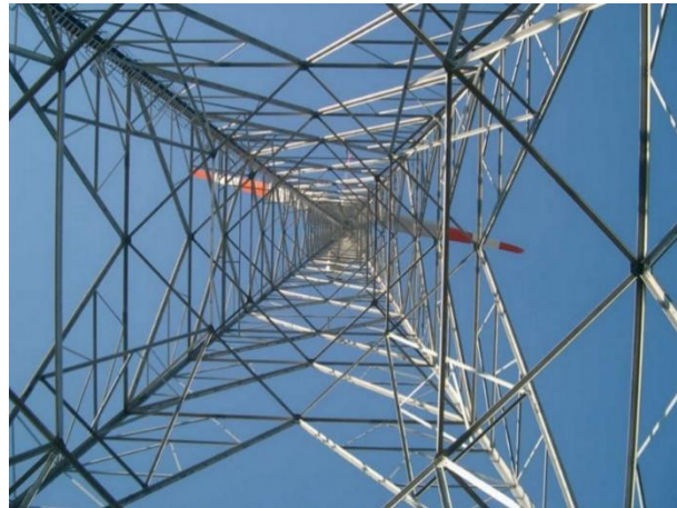
Topview of lattice tower
