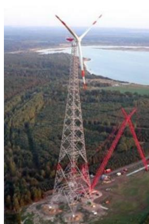
World's tallest lattice tower
