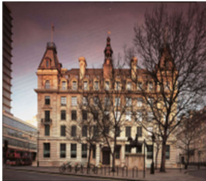
Figure 1.4 Retained façade of Kinnaird House (The free encyclopaedia for UK steel construction information, 2016)
