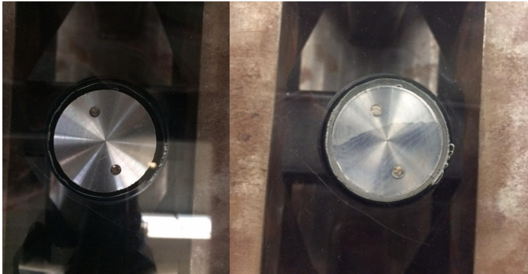
Figure 4.24 Foil-fitting delamination (F1-03)
