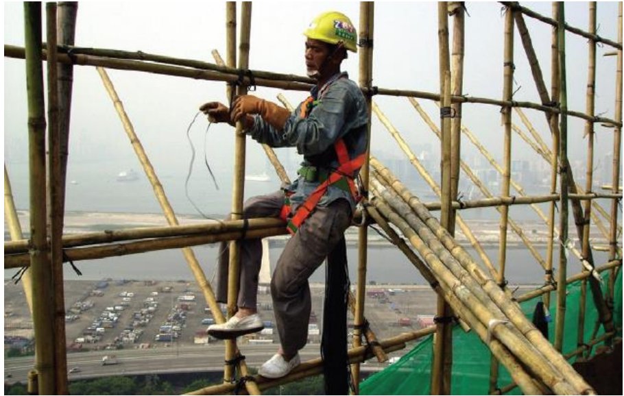
Figure 6.5. Worker Erecting Bamboo Scaffolding [25]
