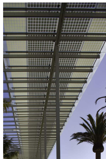
Obr. 3.24: RPBW, California Academy of Science, San Francisco, 2008 - semitrparentní fotovoltaika - www.rpbw.com , foto: Nic Lehoux
