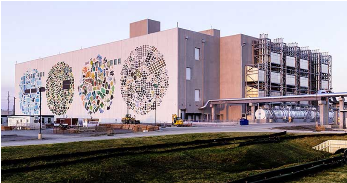
Figure 2.1: A data center building example, Google Inc., Oklahoma.
