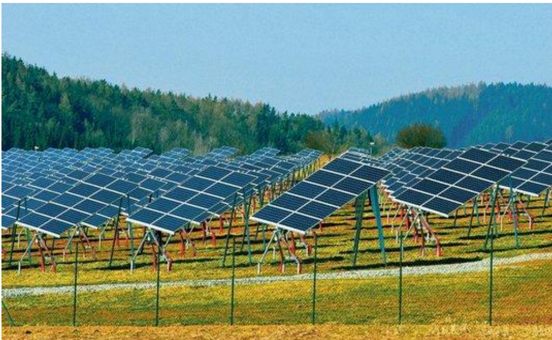
Figure 2.7 - Three Photovoltaic power plants CEZ in Ralsko region
