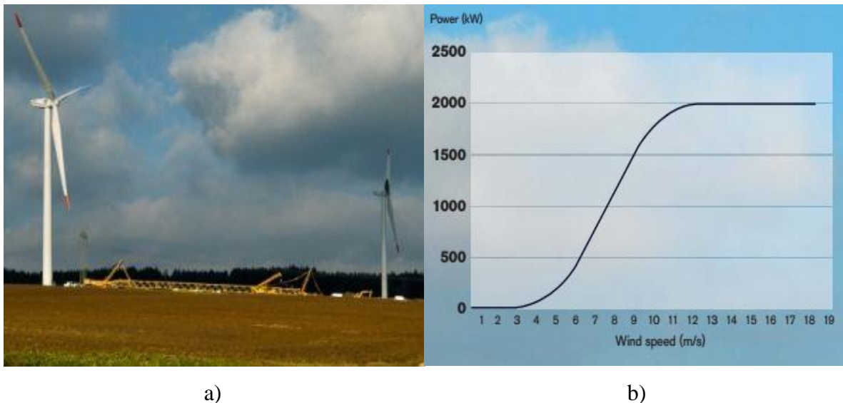
Figure 3.3 – a) Onshore wind power plant in Věžnice, b) The power plant performance
