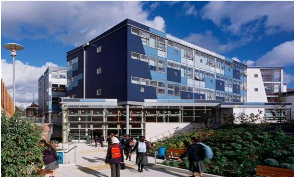
Figure 13: Main academic building of the Bermondsey Academy (Studio E Architects, 2014)
