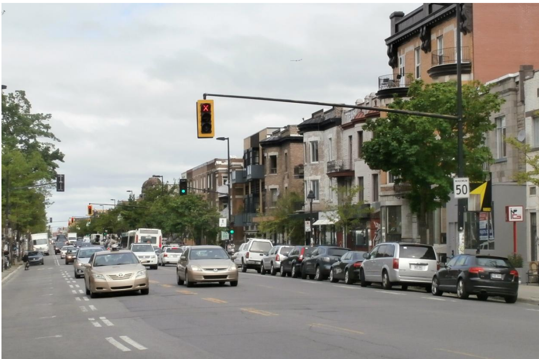
Figure 10: Extra traffic lane with an option of dynamic change of its direction
