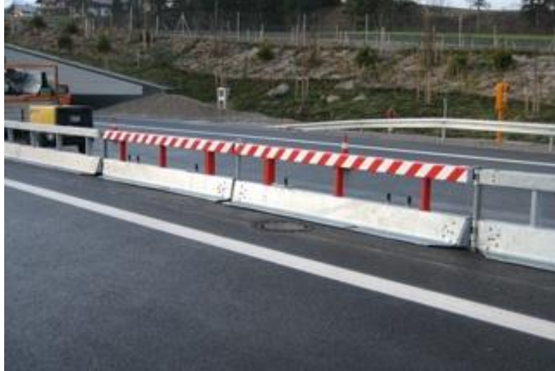
Figure 2.8: Example of an opening safety barrier [1]
