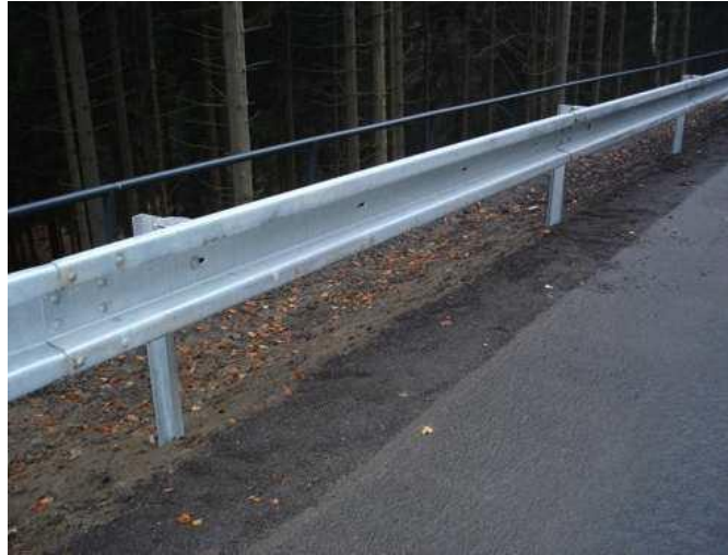
Figure 2.1: Example of a steel safety barrier [42]
