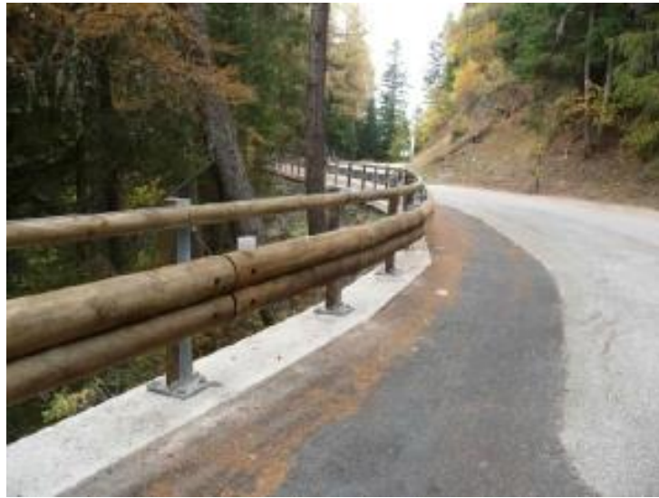
Figure 2.3: Example of a wooden steel safety barrier [41]
