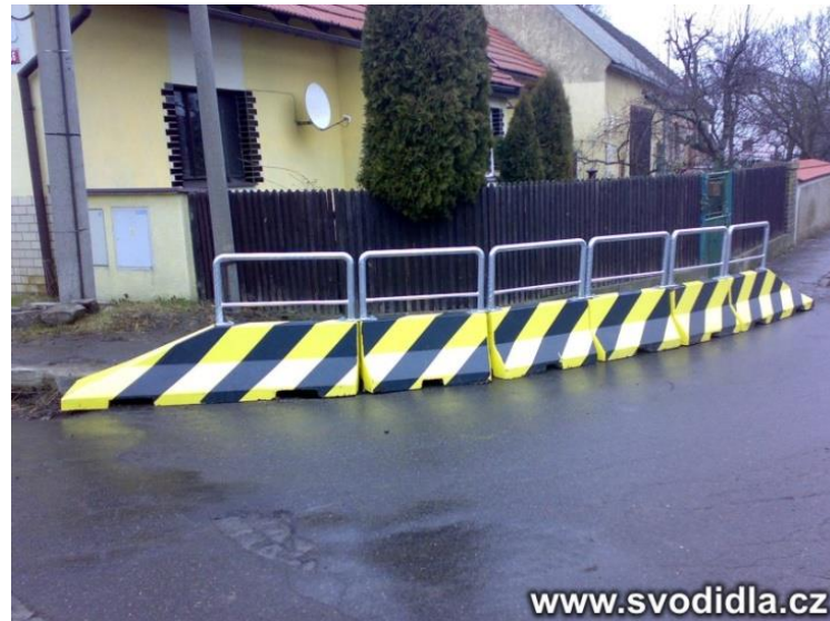
Figure 2.4: Example of a concrete safety barrier [45]
