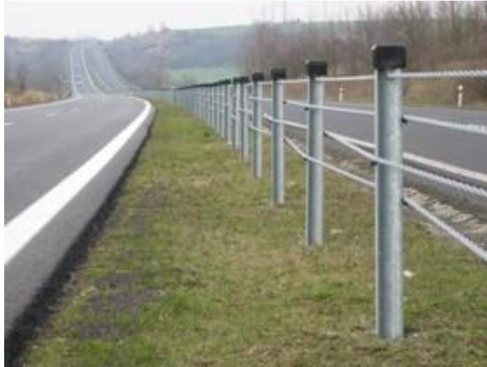
Figure 2.2: Example of a cable safety barrier [37]
