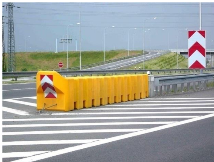
Figure 2.6: Example of a vehicle attenuator [2]
