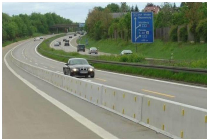
Figure 2.7: Example of a temporary safety barrier [35]
