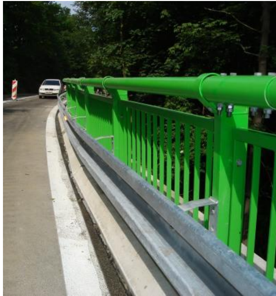
Figure 2.5: Example of a parapet [42]
