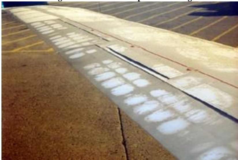
Figure 1 – Hoar frost deposit on a wing
