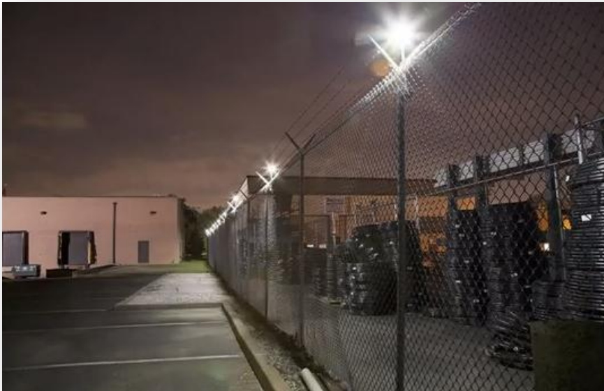
Figure 5: Fenced and enlightened outer perimeter [Source: cast-lighting.com]
