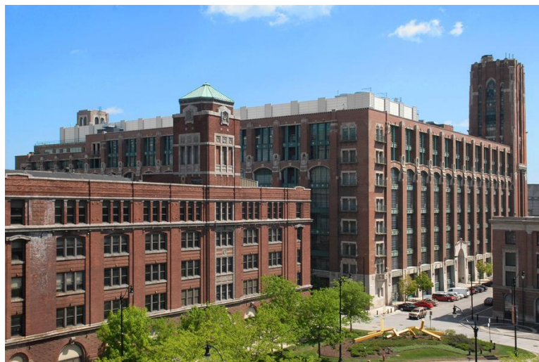
Obrázek 1 - Lakeside Technology Center, Chicago (Forbes, 2015)
