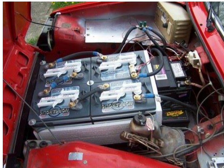
Figure 2-5: Battery pack of lead - acid deep cycle batteries. ( http://www.cbelectriccar.com )
