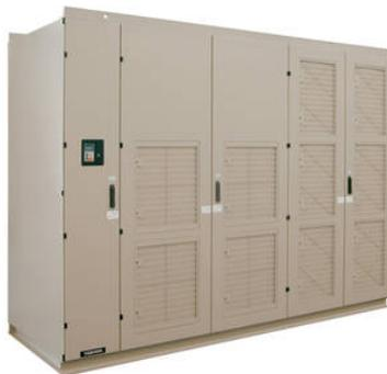
**Figure 1.3.** Medium power matrix converter by Yaskawa
