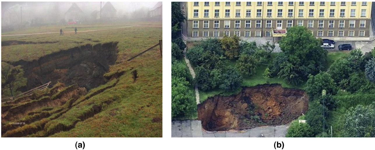
Figure 2.9: Examples of a cave-in collapses, which occurred during construction of tunnels in the Czech Republic: (a) Jablunkov railway tunnel, (b) Blanka road tunnel. Source: www.idnes.cz .
