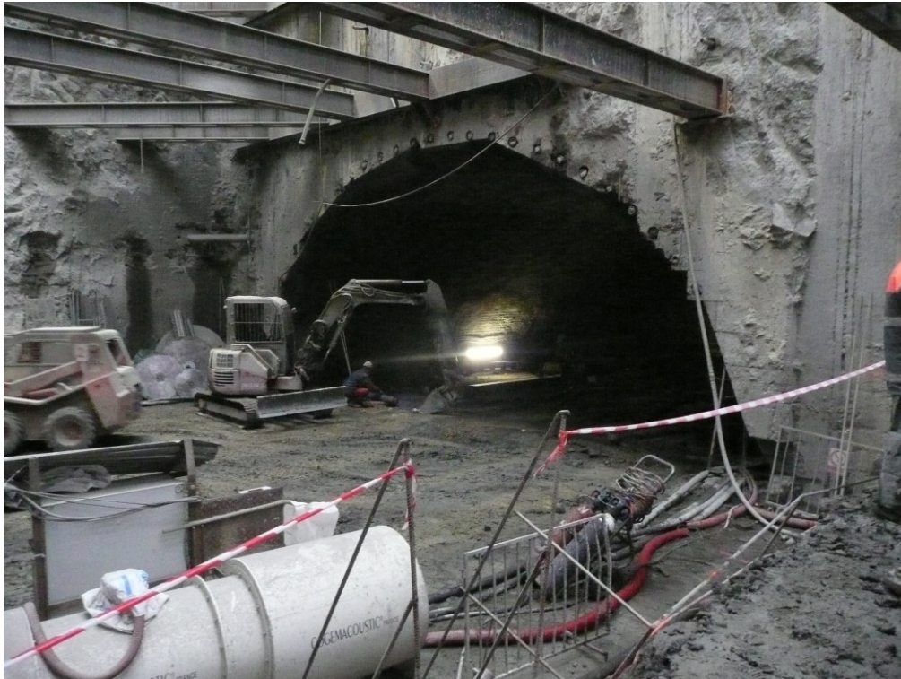
Figure 2.4: Conventional tunnelling in Dobrovskeho tunnel, Brno, Czech Republic.
