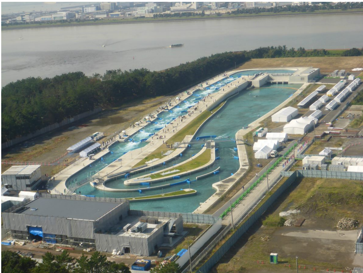
Figure 1. General view of the construction of an artificial riverbed for a wild river in Tokyo.
