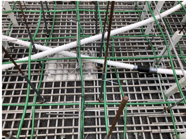
FIGURE 3. Cooling system before concrete casting.
