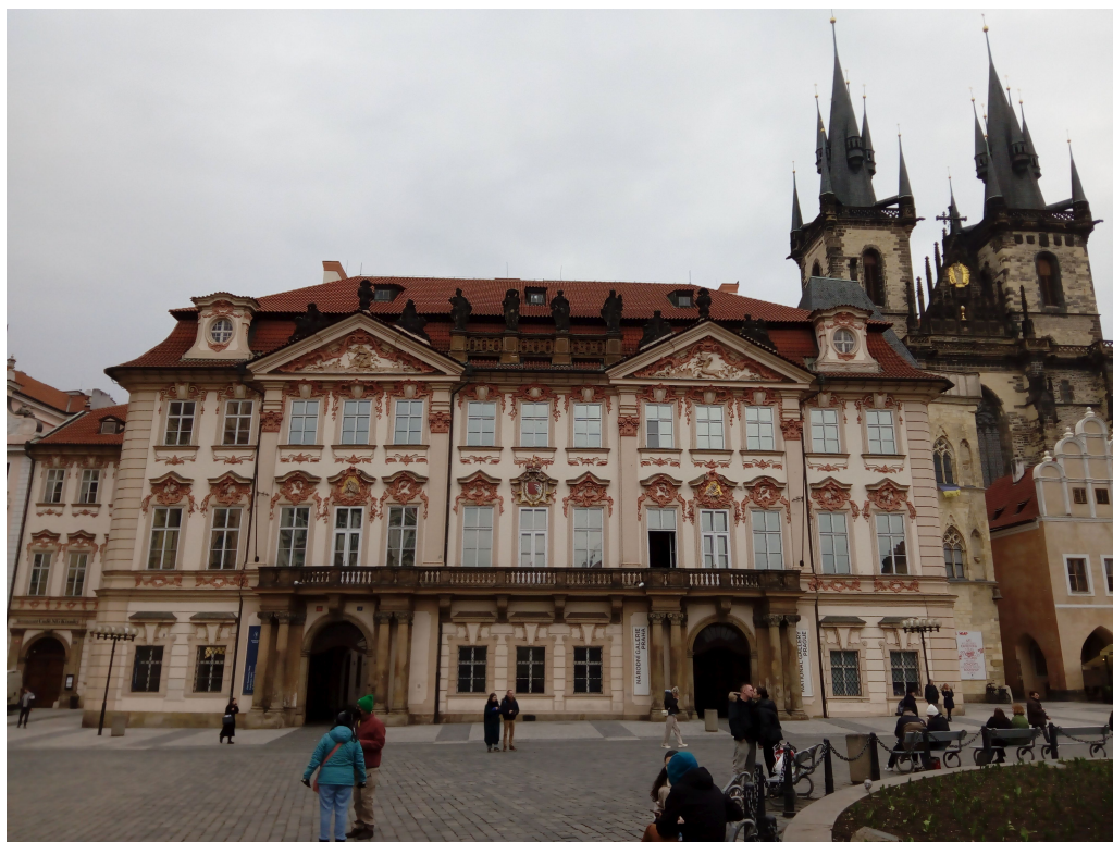
FIGURE 2. Main building of the Masaryk Academy of Labour: Palace of the family Kinský on Old Town Square (1920s).
