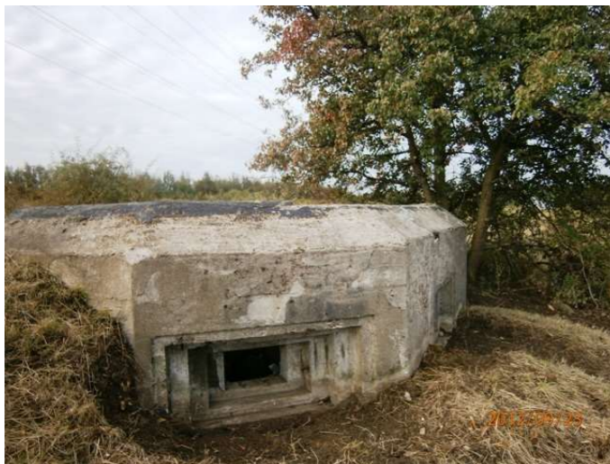
Obr. 49 - Objekt V.b/105/C (Martin Bubela, 2012)
