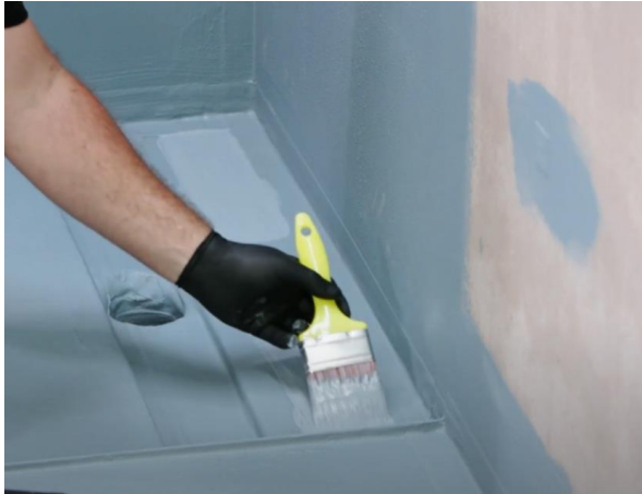
Figure 22: Application of the polymer waterproofing screeds
