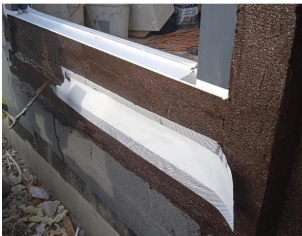
Figure 18: Application of bitumen waterproofing screeds with a reinforcing belt Source: Author
