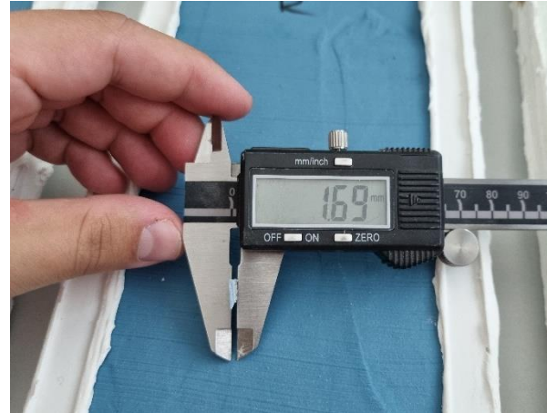
Figure 71. (a) Measuring the thickness of the applied waterproofing screed Source: Author
