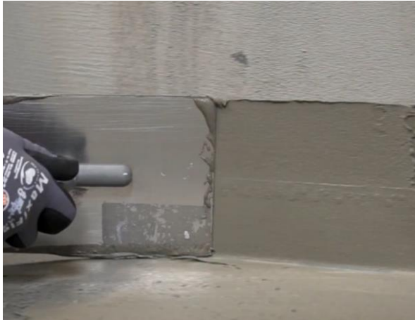
Figure 20: Application of silicate (mineral) waterproofing screeds Source: Author
