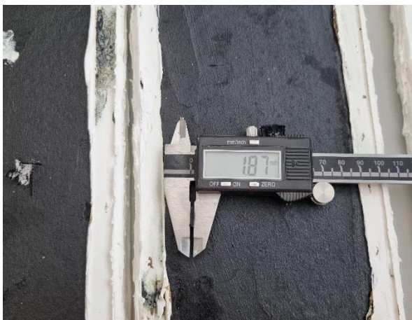
Figure 71. (b) Measuring the thickness of the applied waterproofing screed Source: Author
