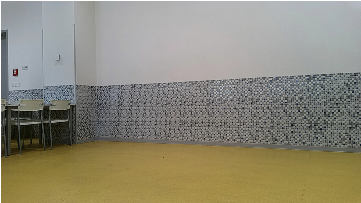
Figure 5.15: A straight wall with a good texture.
