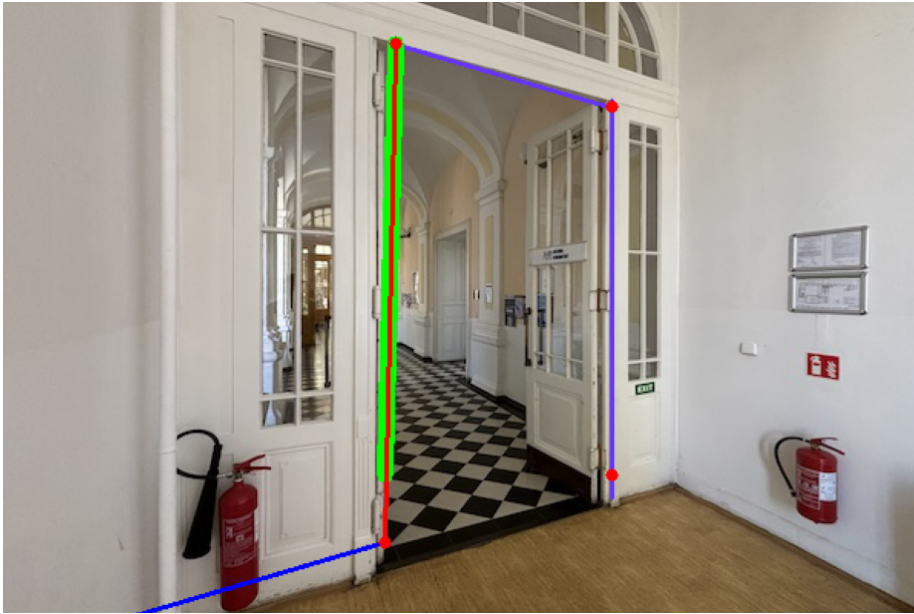
Figure 4.17: Doorway assembly for the 3rd configuration. Green line: door model's left line. Red line: original door's left edge found in the image. Lilac vertical line: doorway's right edge. Lilac horizontal line: doorway's top edge. Blue line: doorway's bottom edge, mirrored from the upper edge.
