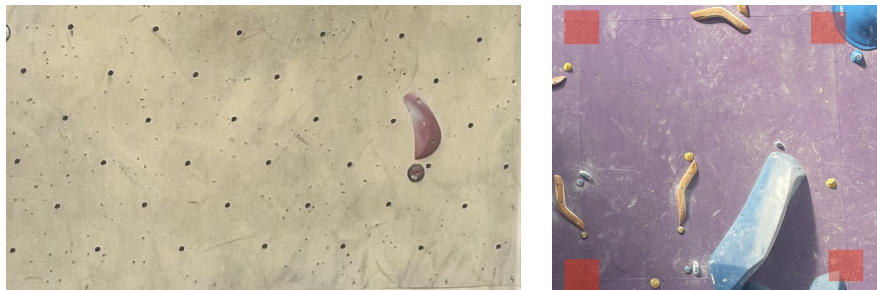
Figure 5.3: Regular elements with known distance. Mounting holes spaced every 20 cm diagonally (L), and square panels of dimensions 100 \times 100 cm (R).
