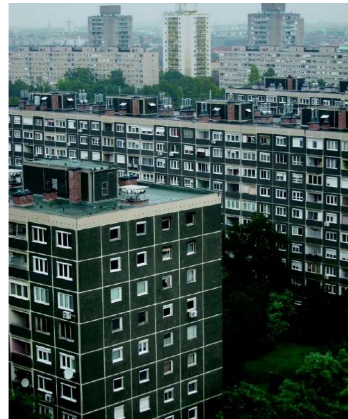
Kelenföld, Budapest: pioneering prefabricated blocks built from 1965 using a Soviet spin-off of the Camus system. Source M Glendinning, 2015
