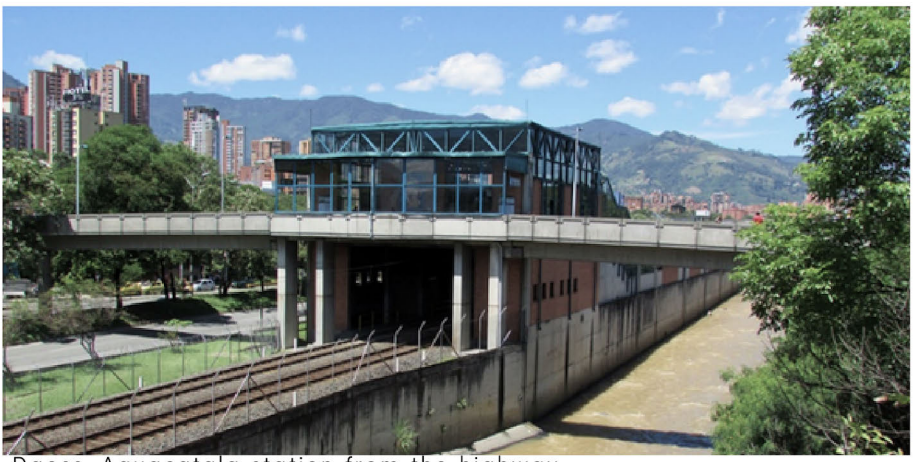
Daoss, Aguacatala station from the highway
