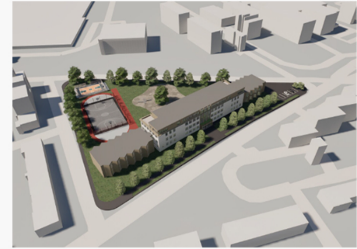
The final form is a combination of a 4 level volume, the new added floor and volumes is being made of aluminium panels to visually separate of the rest of the building
