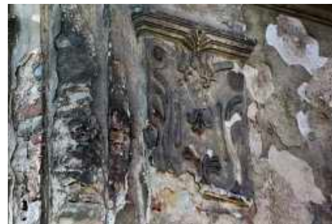
SV04 Obr. 1: Detail fasády, 1976
