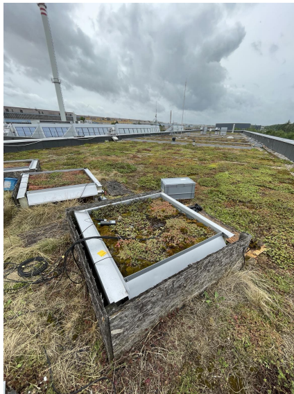
Figure 29: Experimental green roof area
