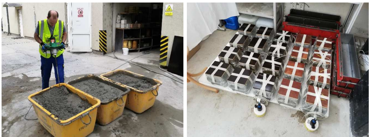
Figure 70 - Mixing of adapted concrete batches, early-age compressive strength samples [photo: author]
