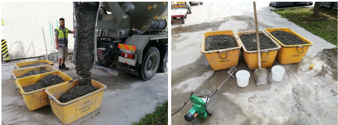
Figure 69 - Preparation of concrete batches, three concrete batches before adaption [photo: author]
