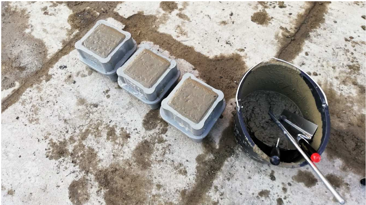
Figure 14 - Cube sampling on the construction site [photo: author]
