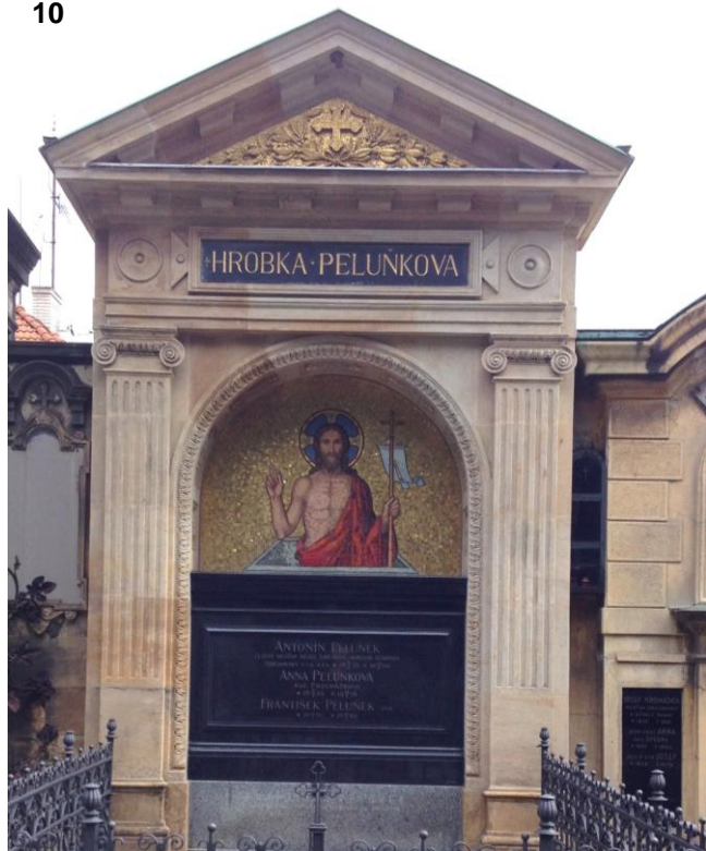
Peluněk Family sepulchre after restoration.
