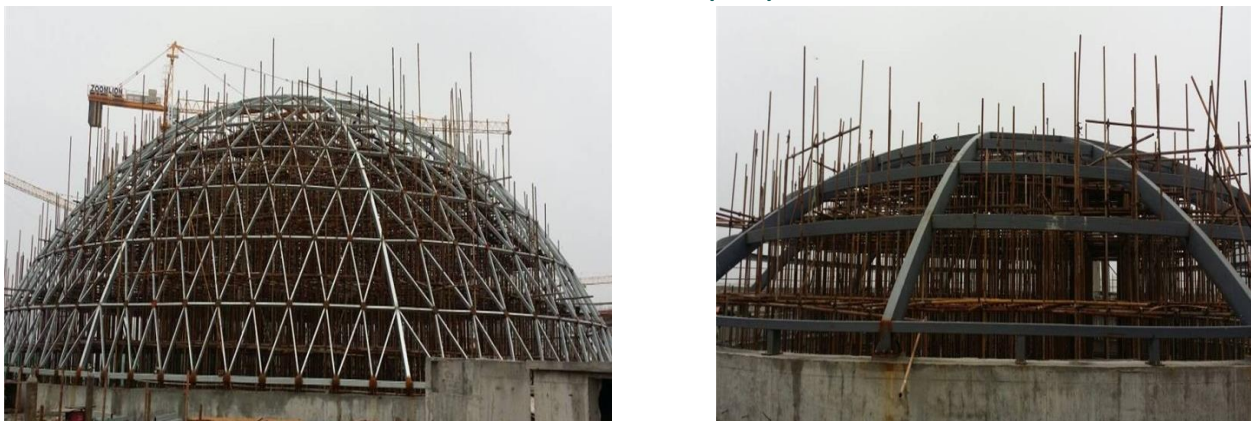
Figure 1.2 Examples of RHS application in dome welded truss steel structure roofs (China)
