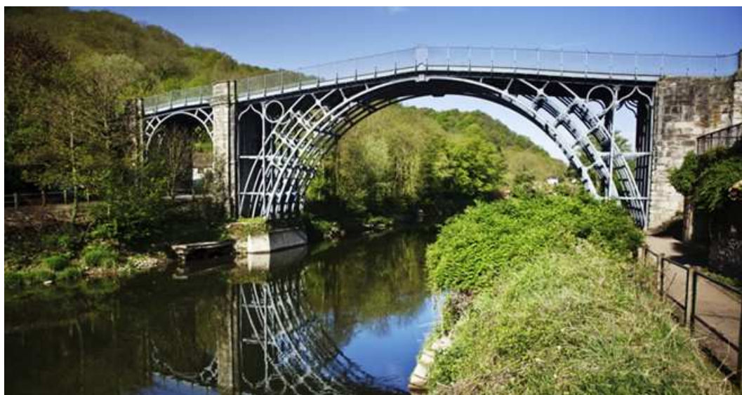
Obrázek 8 Iron bridge, Shropshire [19]
