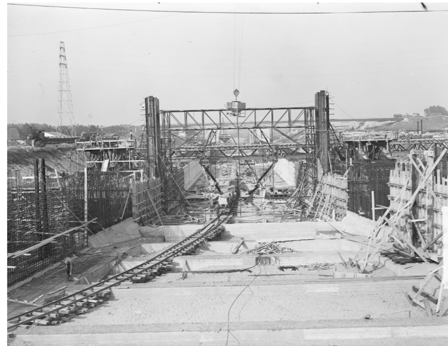
Lock building in Tiel in Amsterdam-Rijnkanaal Date: 13 October 1949
