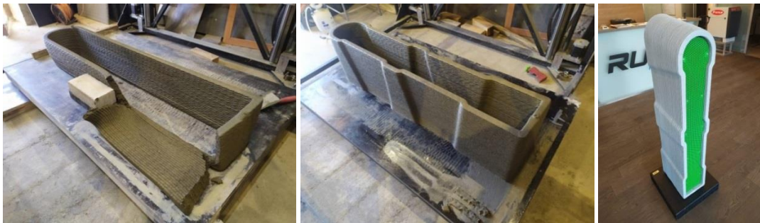
Fig.81. a) Collapse of the wall of charger version A printout during printing due to buckling b) Successfully completed printing of the charger body version B after modification of the model and insertion of stiffening elements
