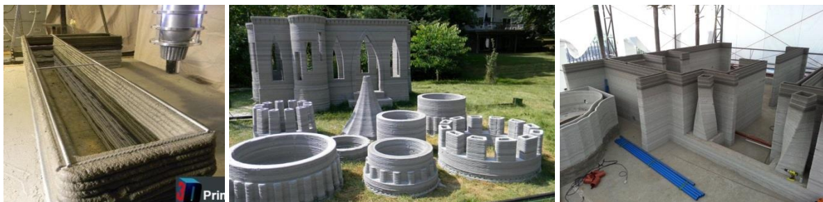
Fig.10. 3D printing at Total Kustom, USA a)Printing process b) Printed part of a castle c) 3D printed hotel in Phillipines in progress
