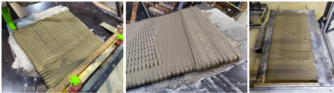
Fig.69. a) Test of 3D printing on inclined board using angled nozzle b) Detail of the panel end showing the change in layer thickness due to the increase in pump pressure c) Printout of panel 3
