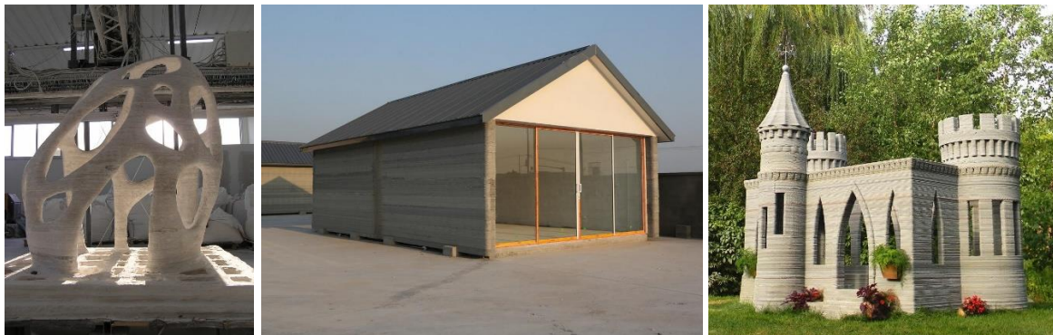
Fig. 1: a) Radiolaria pavilion developed by Andrea Morgante of Shiro Studio and 3D printed by D-Shape technology b) Simple building, made of 3D printed walls by WinSun technology c) Model of a castle, made of 3D printed parts by Andrey Rudenko, TotalCustom
