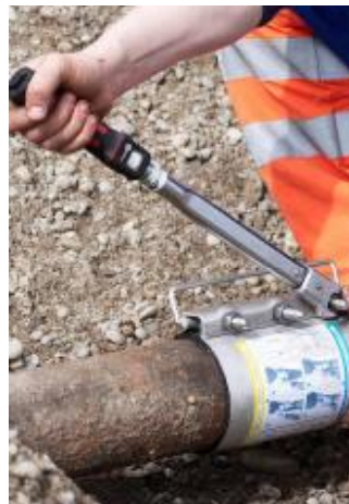
Fig. 1: Tightening of the joints by a torque wrench (Cézová, 2017).
