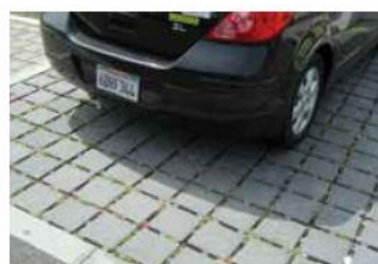
3 Stormwater is infiltrated through the use of permeable paving systems, landscape planters and other purposely located pervious surfaces.
