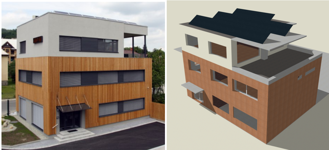
Figure 13.2.: Fenix building. Credits :Fenixgroup, Miroslav Urban
